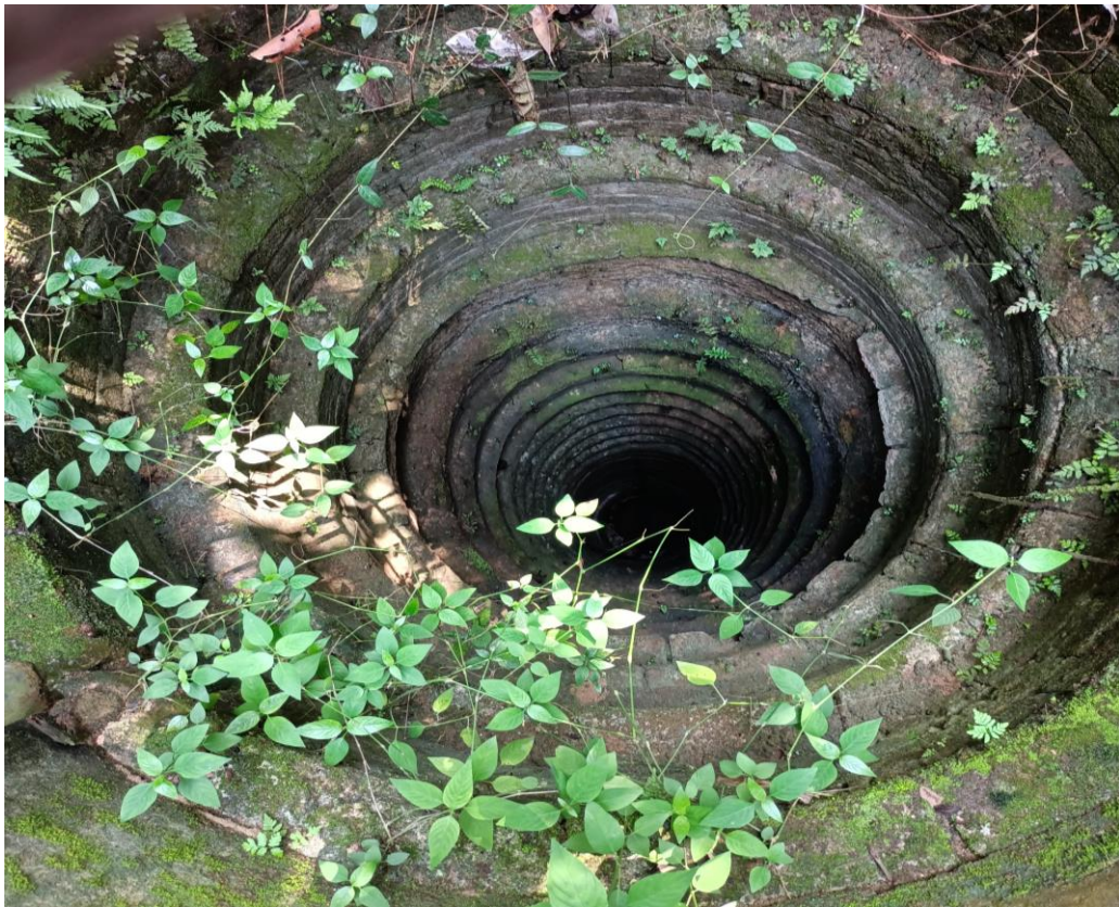
Photo 5: Dried well at Thonnakal due to clay mining activities.
